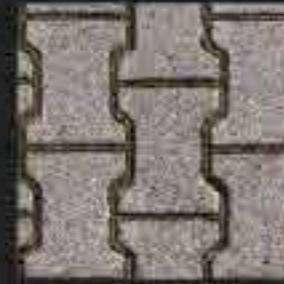
INTERNAL ROADS INTERLOCKING BLOCKS/ TREMIX CONCRETE ROAD
