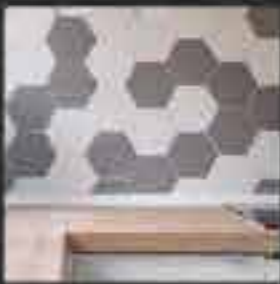
DADO CERAMIC TILES 600 MM ABOVE THE COUNTER
