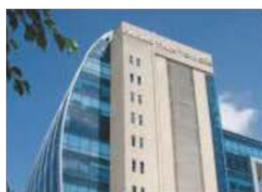
PARAS TWIN TOWERS
